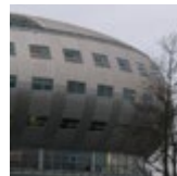
HOLLAND Hot water pumping across district network
