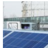
ITALY Cooling loop flow & temperature control
